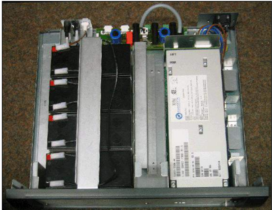
Figure: OpenScape Business Powerbox – Equipped with four 12V 7Ah batteries and LUNA2 power supply
